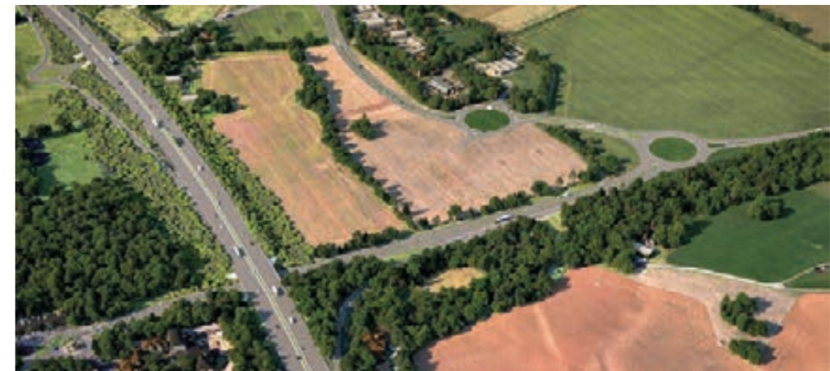
▲ Improved motorway junction
