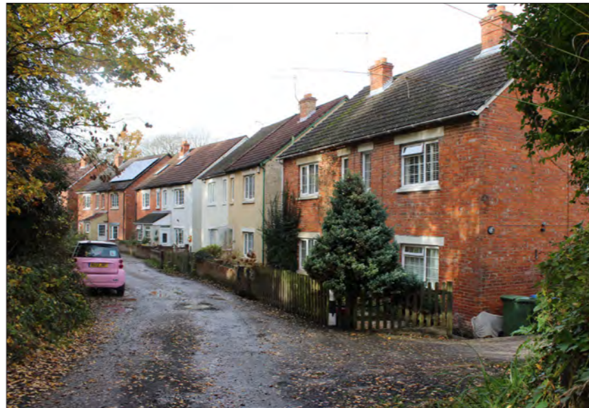
Some of the Victorian red brick houses that still remain at the core of Funtley.
