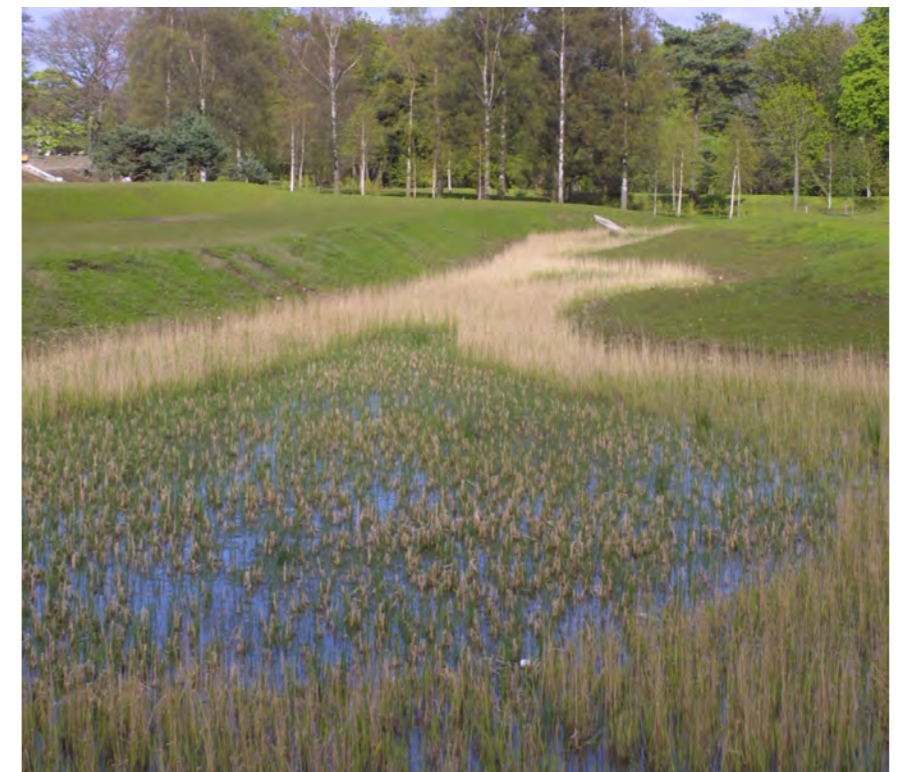
Retention basin, a SuDS component
